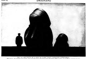
FIG. 11.—BUCKETS OF 5 AND 54 CUBIC FEET CAPACITY COMPARED.
